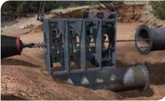
Fig. 1: Steel Cable and Roller Reduction Box
