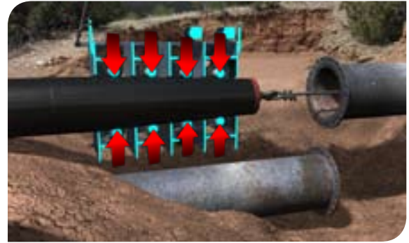
Fig. 2: Hydraulic Rollers
